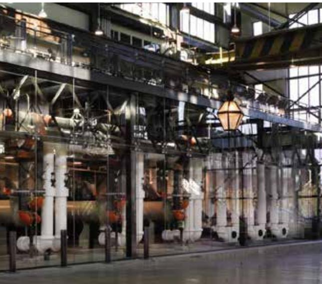
At this retailer's headquarters, a 3,400-ton central plant was constructed and installed with three chillers and all associated equipment. The new and improved system provides more efficient operation and dramatic energy cost savings to the entire headquarters campus.
